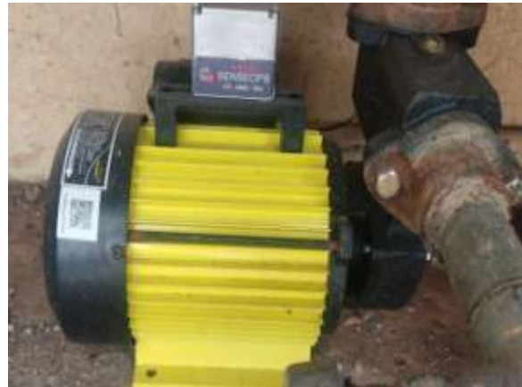
Fig 5. Sensor mounting on AC induction motor.
