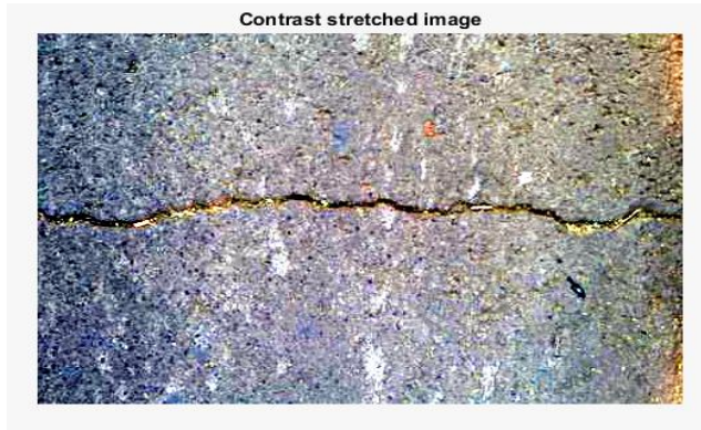
Fig2: Contrast Stretched Crack Image.
