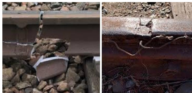
Fig. 1 Cracks on railway track
