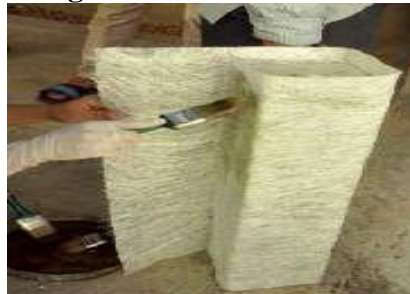
Figure 9:Wrapping of GFRP Mat
