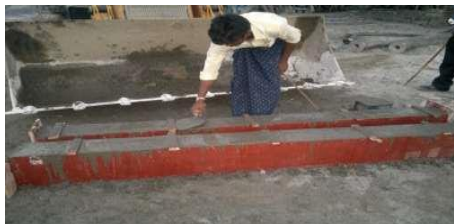
Figure 3: Casting of Beams
