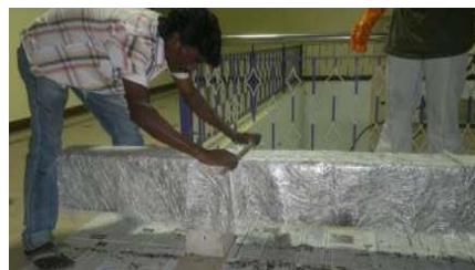
Figure 6: Rolling after U Wrapping GFRP mat for Beam S-1
