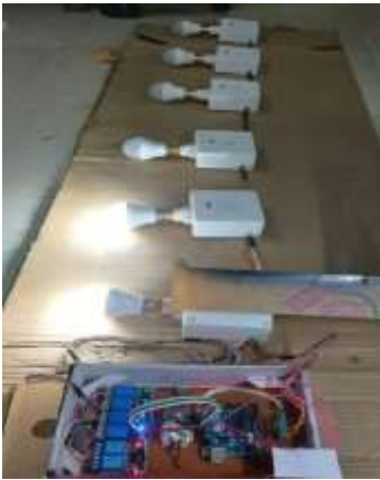
Figure 5. Operation Phase 1 of street light automation
