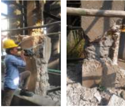
Fig.1. Removal of existing plaster
