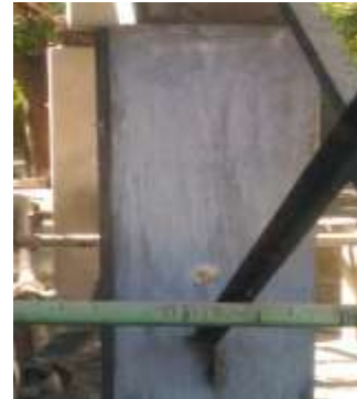
Fig.4. Concrete jacketing
