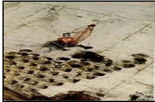
Fig-3 Deep dynamic compaction
