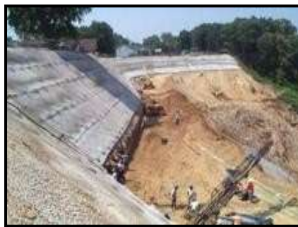
Fig-14 Soil Nailing
