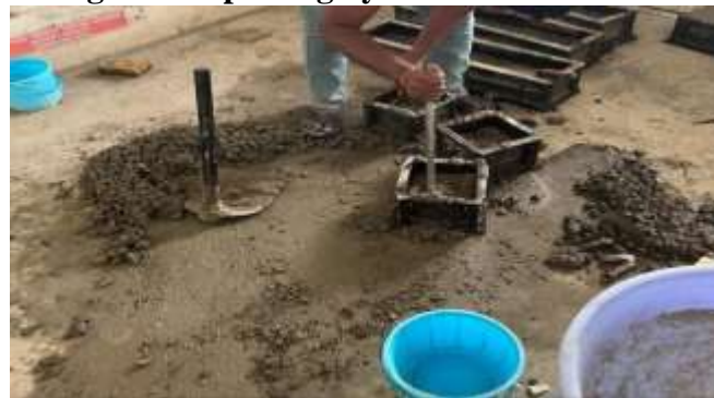
Fig: 5 Compacting by hand
