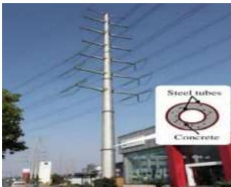
**Fig 1.4: Application of CFST column as a powerline pole**
