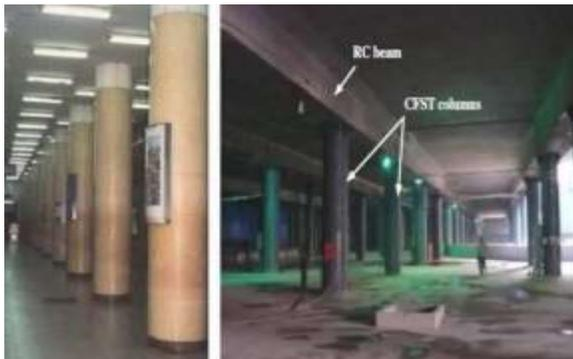
**Fig 1.3: Application of CFST columns in buildings**
