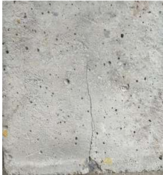
Fig 2.4 Shows the specimen after pre-cracking
