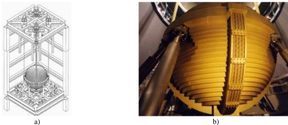
Figure 1 – Taipei 101: TMD general configuration (a) and primary viscous dampers (b).
